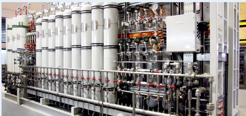
Wellhead Control Panels / Hydraulic Power Units
