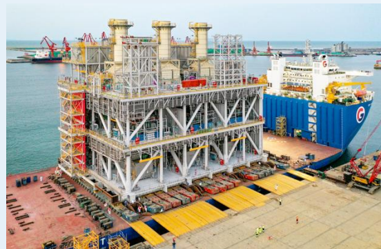
Waste Heat Recovery Units
