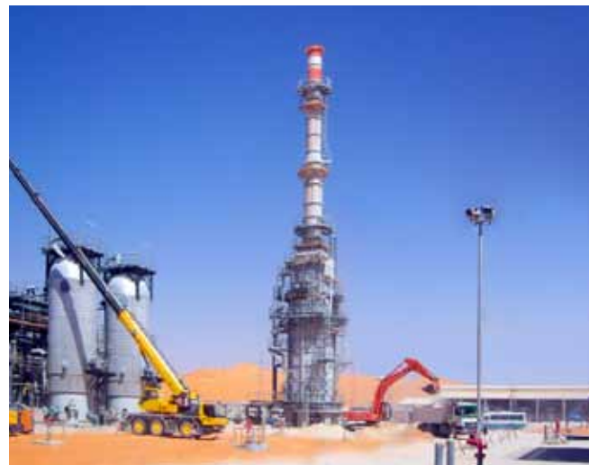
Regeneration gas heater, Algeria
