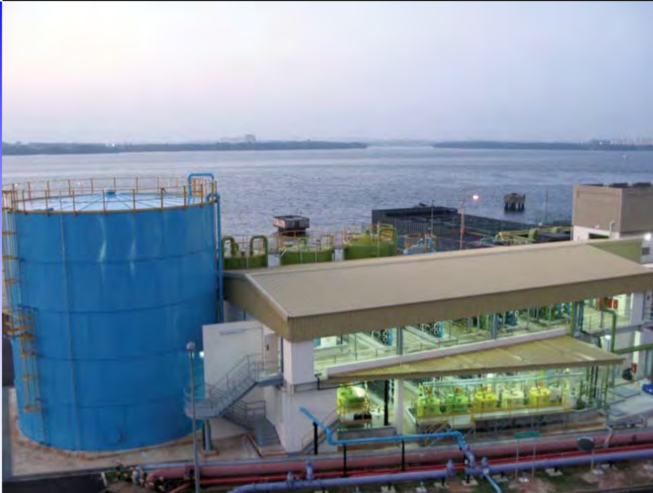
Senoko Power Seawater Desalination Plant SINGAPORE
