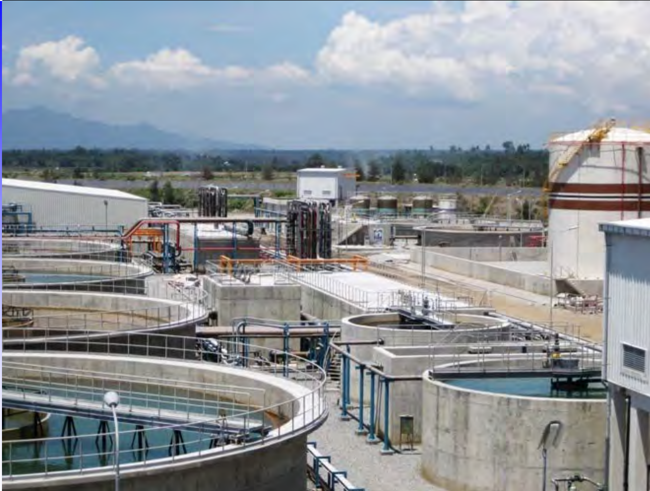
Tanjung Jati B Seawater Desalination Plant INDONESIA
