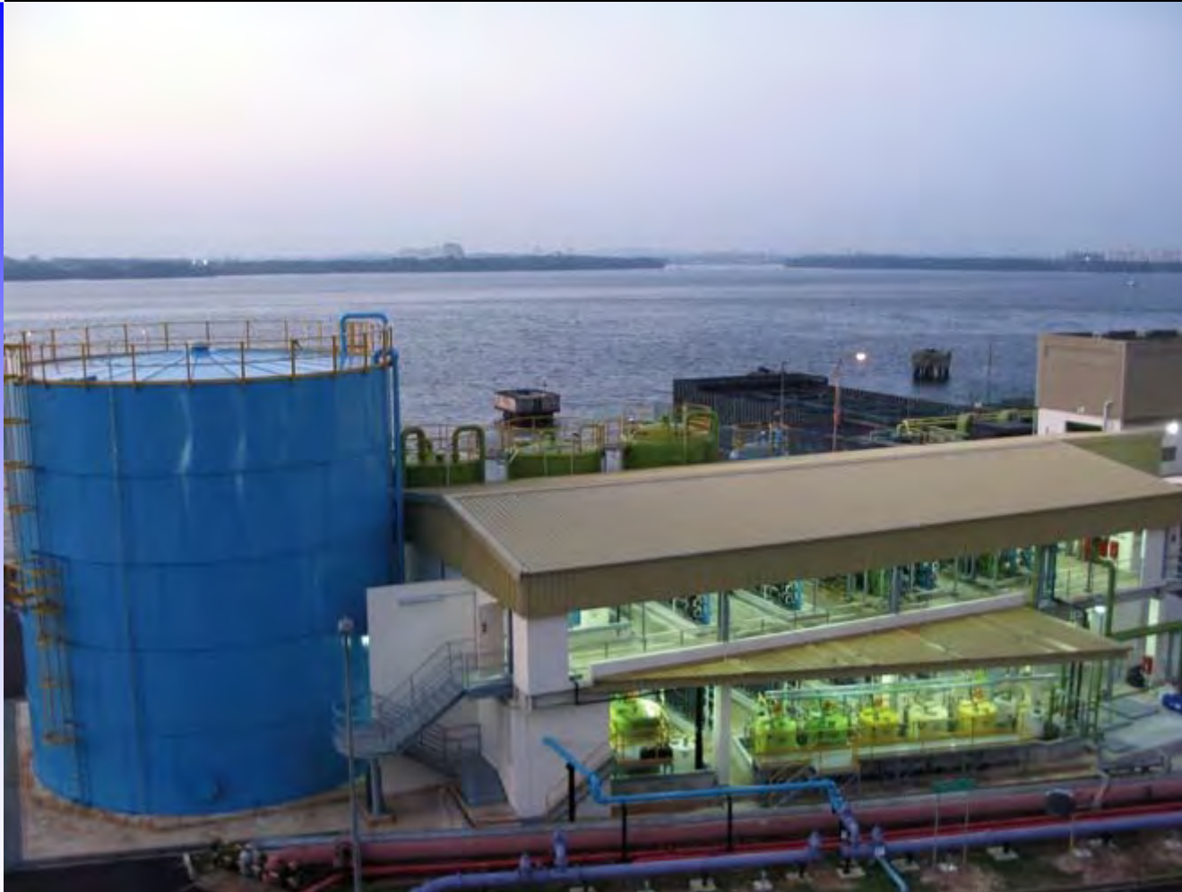
Senoko Power Seawater Desalination Plant SINGAPORE
