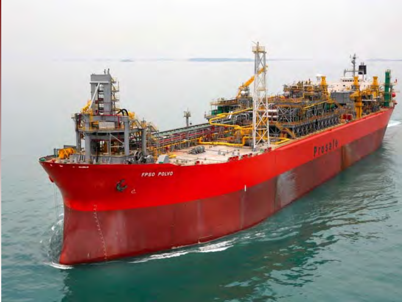
ICSS system onboard FPSO Polvo BRAZIL
