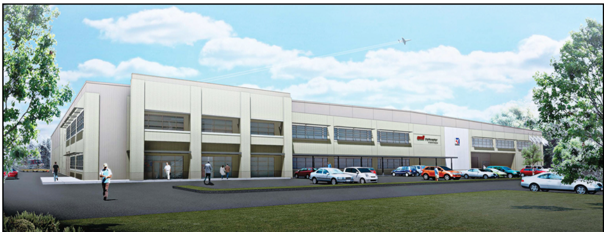
Artist's impression of 15,000 sqm MRO hangar facility to be completed by 2Q 2012 *
